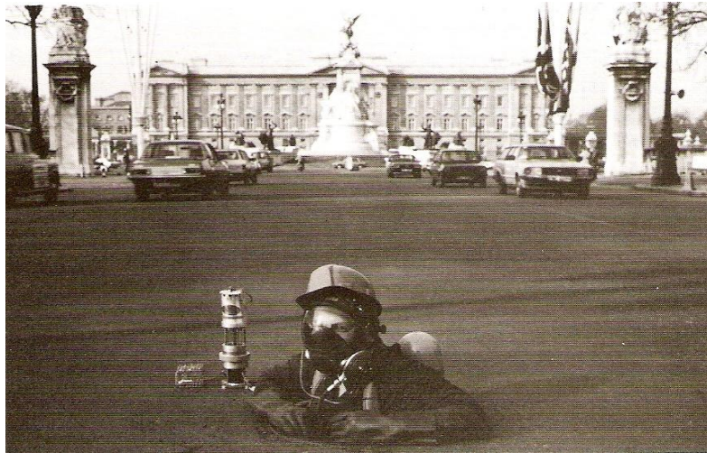
Figure 20: The Sewer running through the Buckingham Palace (Trench and Hillman 1985)
