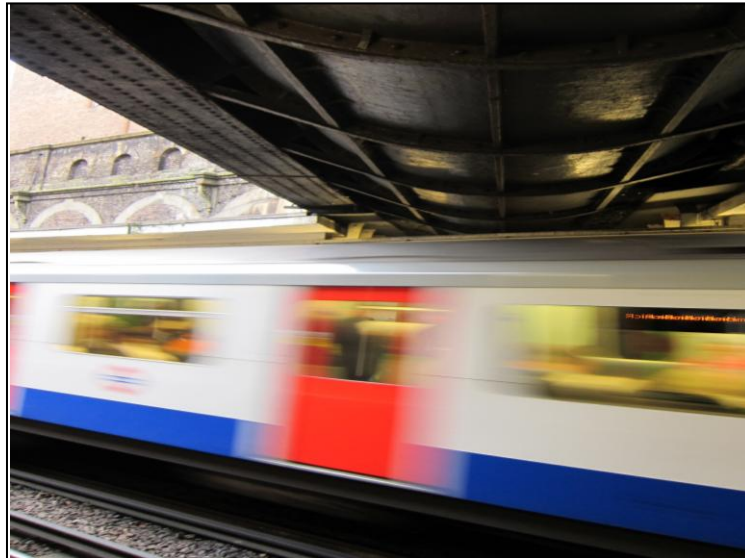
Figure 8: The Kilburn flowing above Sloane Square Tube Station in a cast conduit
