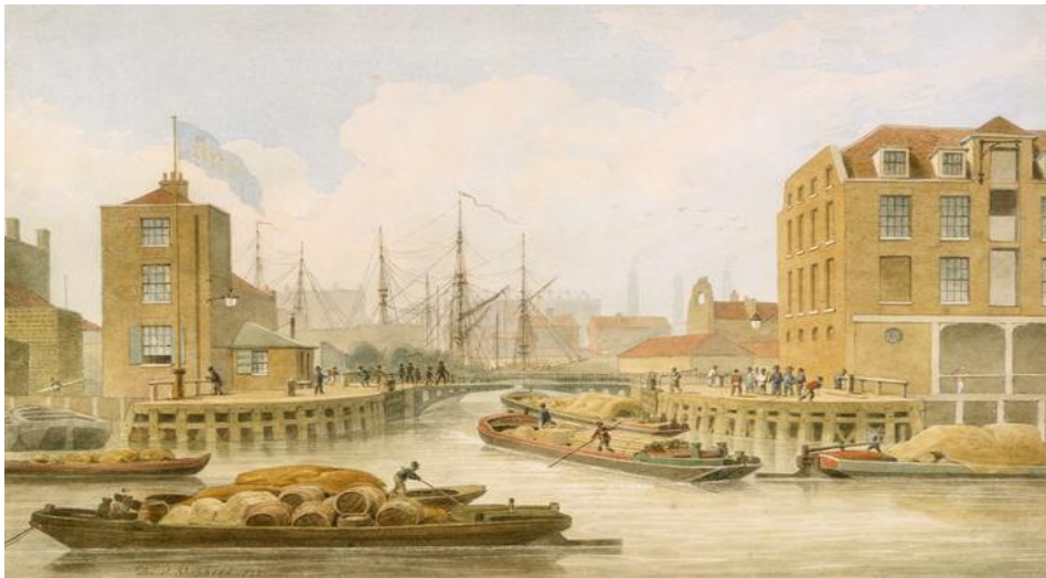
Figure 14: Barges entering the Regent's Canal at Limehouse from a watercolour (London Metropolitan Archives 1823)
